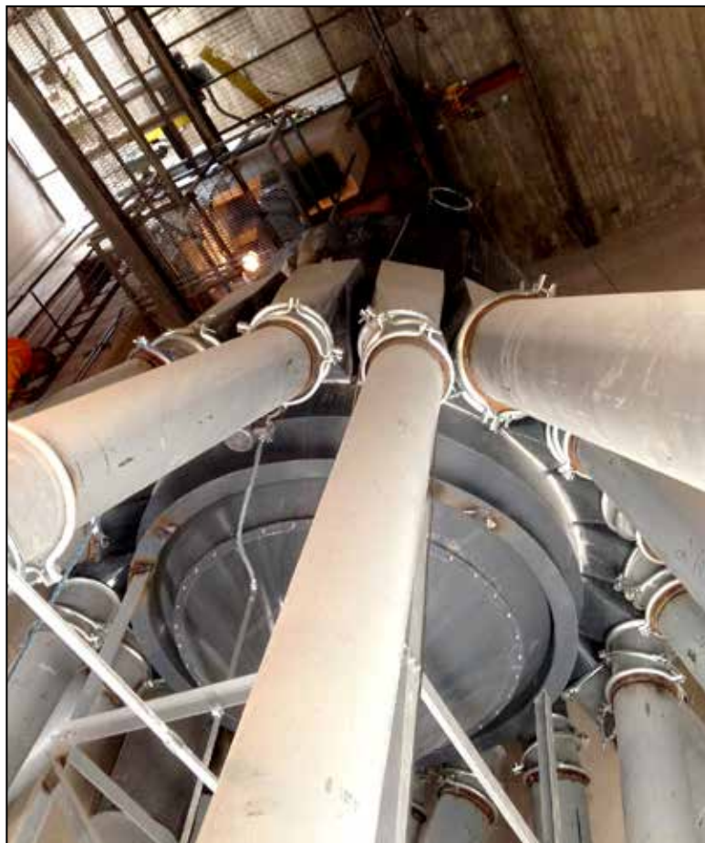
PICTURE OF THE NEW DISTRIBUTOR IN THE HEAD HOUSE
